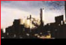
Enron's 116-megawatt Elektrociepłownia Nowa Sarzyna cogeneration power plant was the first private, independent power project in Poland, and one of the region's first natural gas-fired, cogeneration plants.
